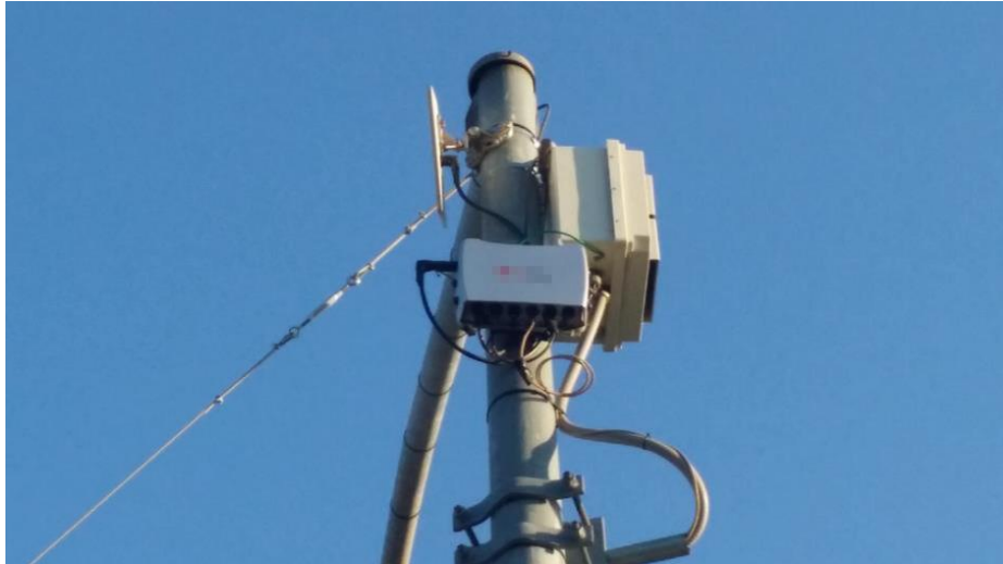
Figure 1: The security system
