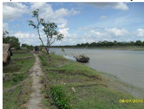
Plate: Earthen Levee along the Maidara river to prevent tidal intrusion in the Project area
