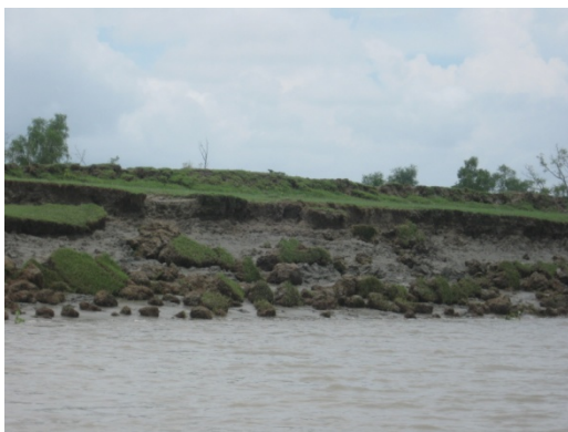
Plate 6.1: Erosion at right bank of the Passur River (Chunkuri village)
