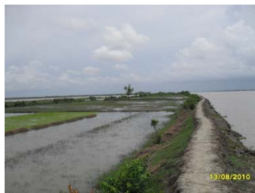
Plate: Earthen Levee along the Passur river to prevent tidal intrusion in the Project area
