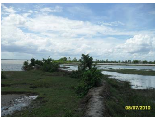
Plate: Earthen Levee along the Passur river to prevent tidal intrusion in the Project area
